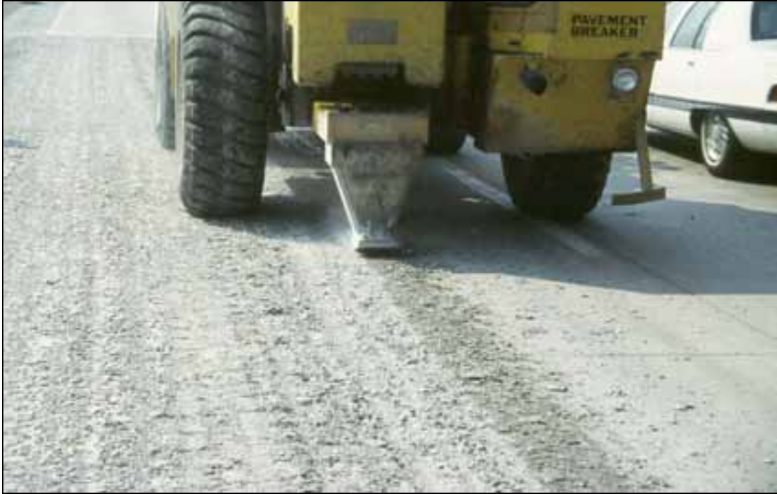
Figure 2.4 Resonance Frequency Breaker (Photo courtesy of Dr. Kevin Hall, University of Arkansas).
