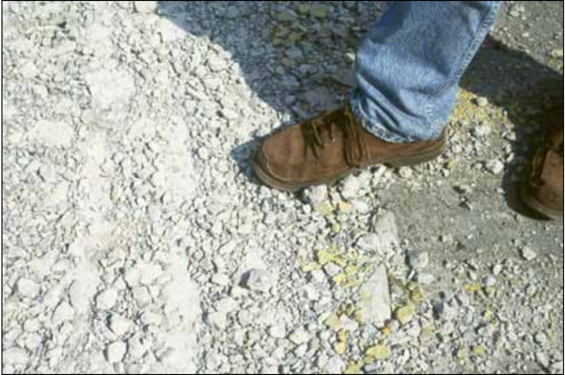
Figure 2.3 Rubblized Pavement.
