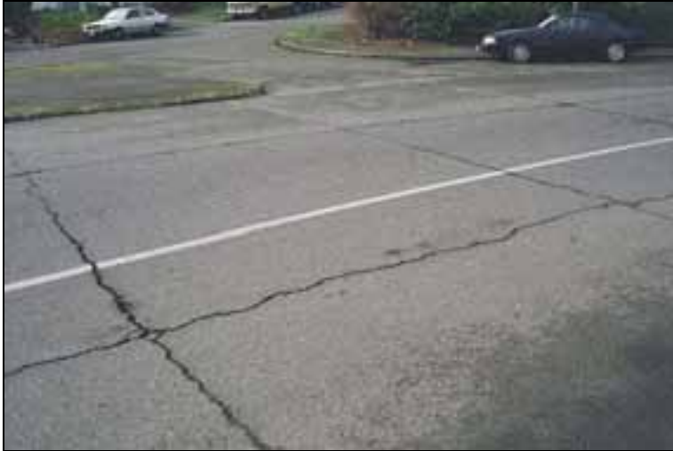
Figure 2.1 Reflective Cracking.
