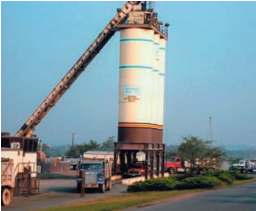
Superior Paving Corp.'s Leesburg Plant
